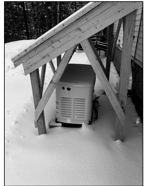
A newly installed GENERAC 22 Kw generator at American Legion Cecil R. Cole Post 94 provides power in the event of long-term outages.
