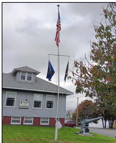
Flying Again After The Storm: The flagpole at Post 35 is back to its operating glory after minor damages from Hurricane Lee.
